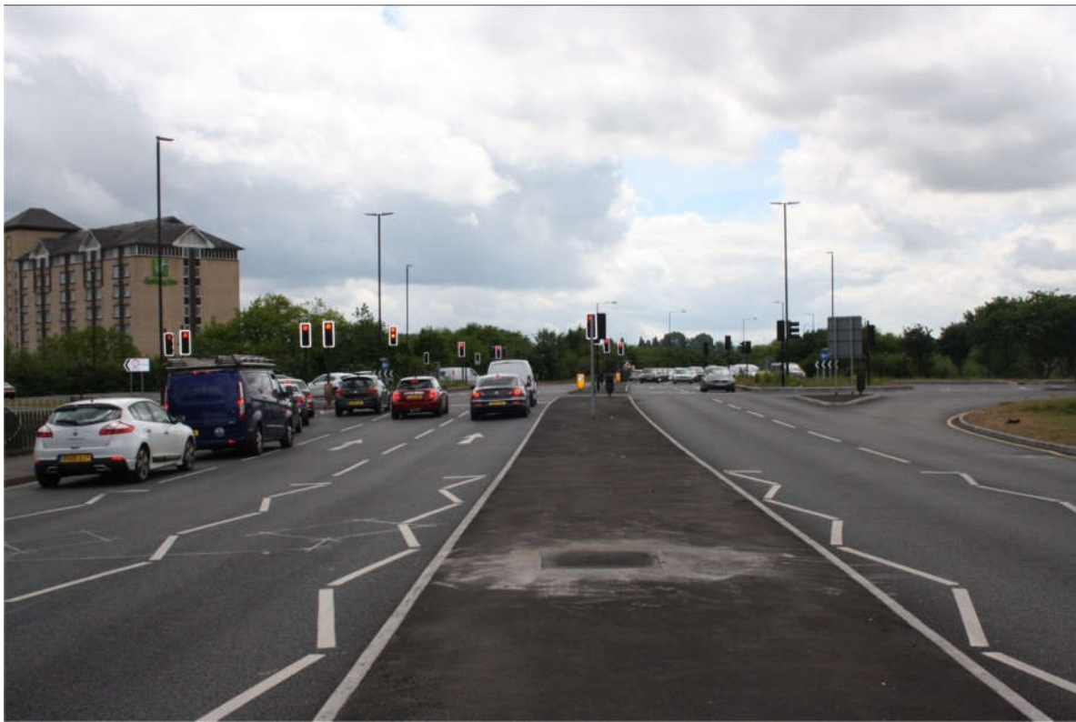
Figure 1 A355 southbound approaching Copthorne roundabout
